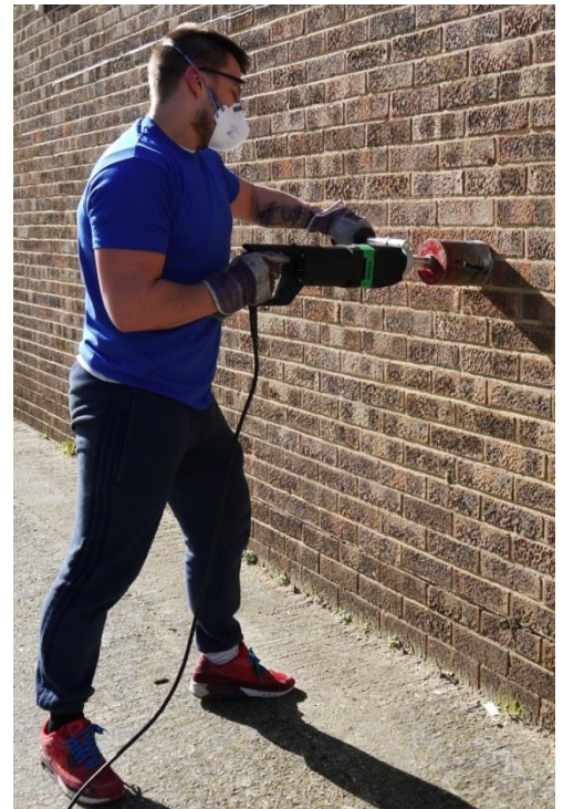
CORRECT DRILLING POSITION
